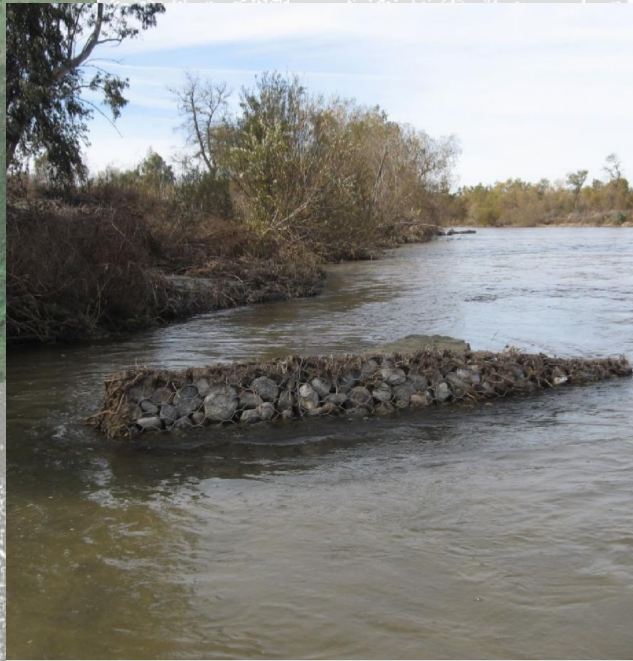
Rock gabion 9 months after installation
