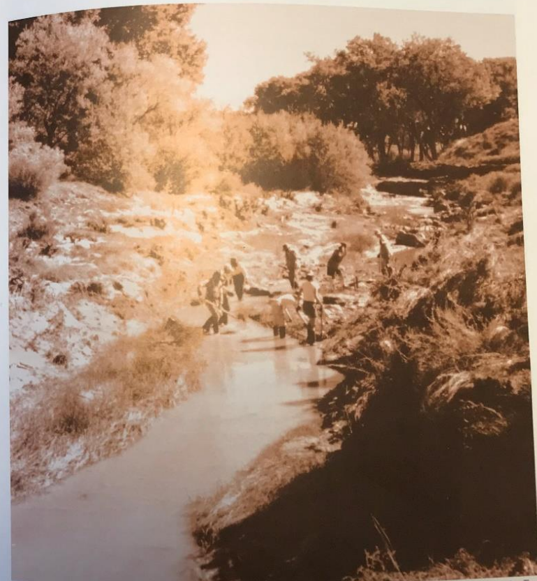
Volunteers construct small water-diversion structures within Pueblo Colorado Wash to encourage the formation of stream meanders. The work is part of a three-year demonstration restoration project at Hubbell Trading Post National Historic Site.
