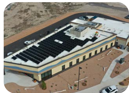
Aerial view of the Confluence Center and its rooftop solar array.
