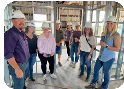
RiversEdge West staff tour the Confluence Center while under construction.
