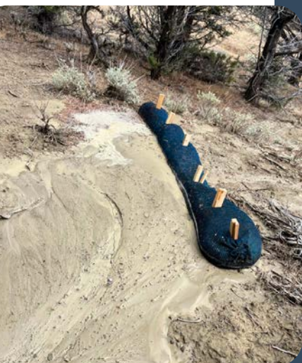
Wood wattle in action at Jumbo Mountain during a storm event.
