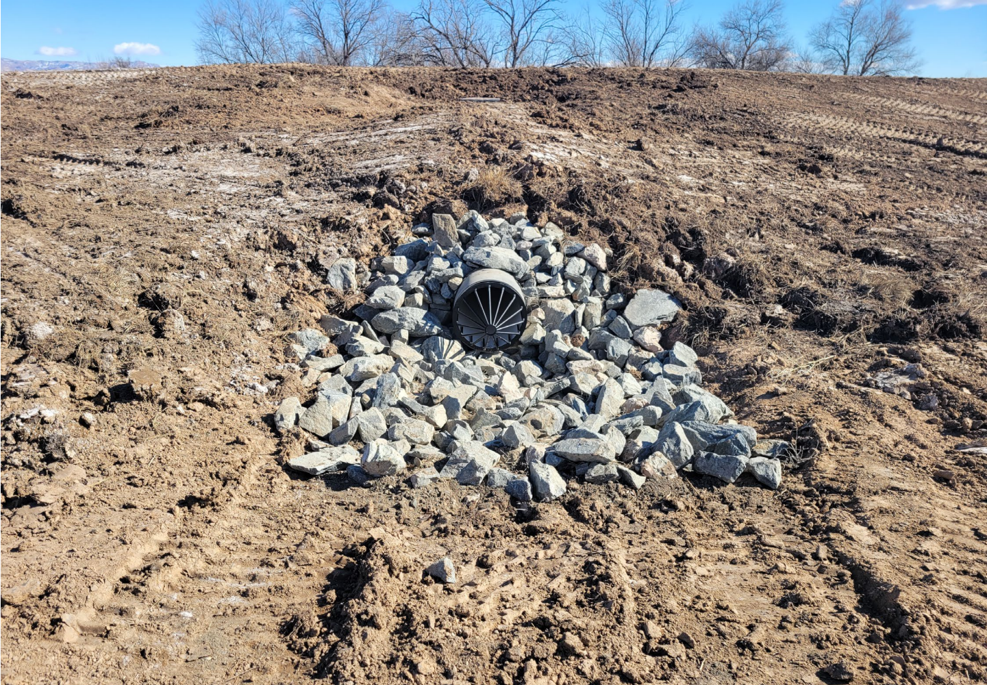
Agri-drain buried in embankment
